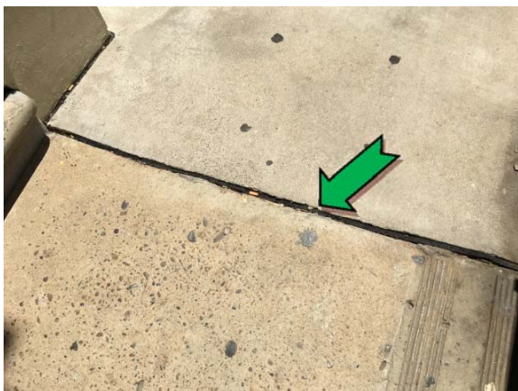
Photo 5. Exterior, throughout, ground, expansion joints – suspected non asbestos-containing construction mastic.
